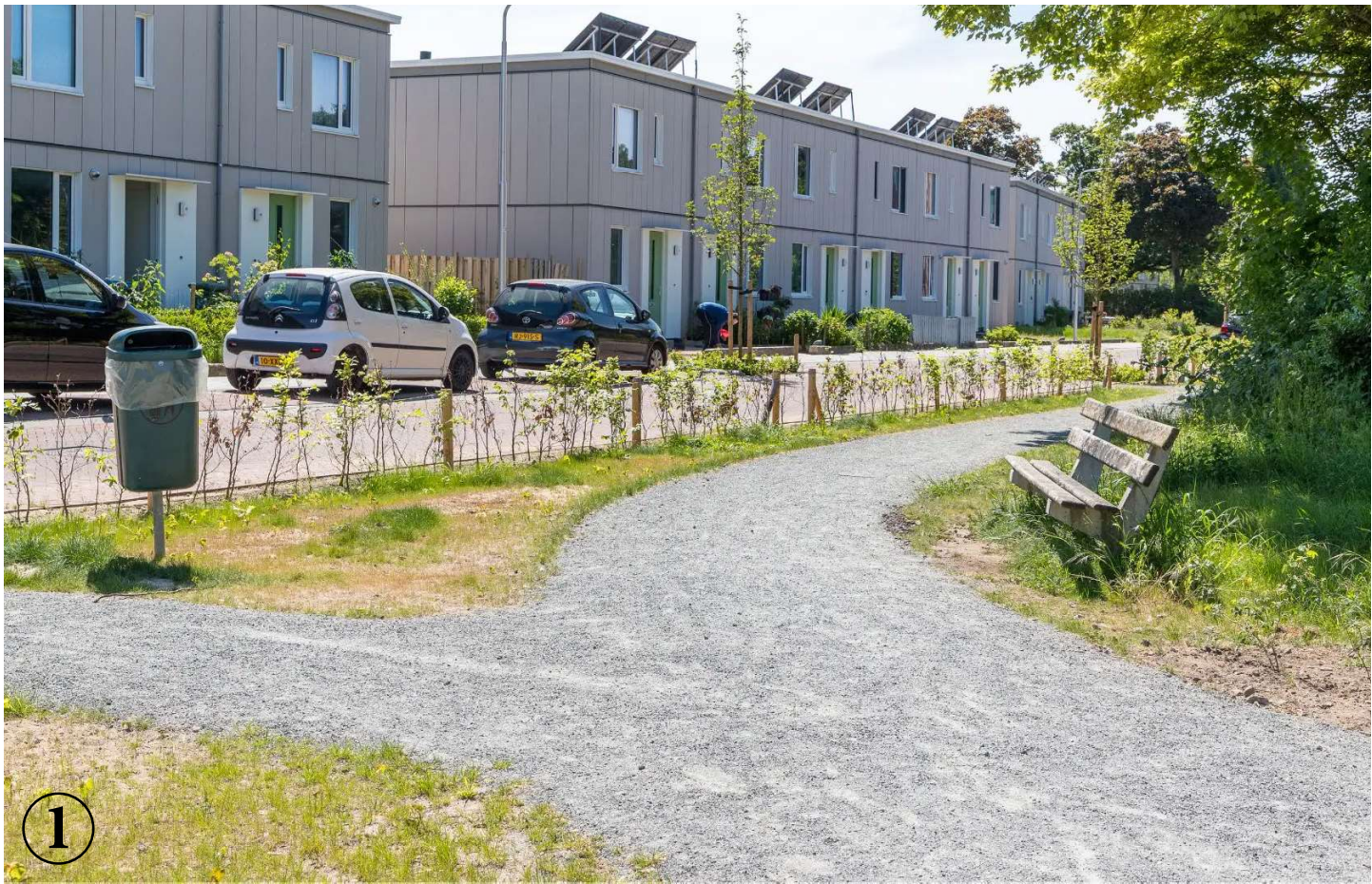
halfverharding waterdoorlatend, maar rolstoel-proof, route oost-west
